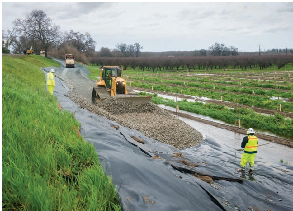
A Delta levee being repaired.
